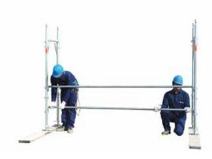
6 • erecting the second ledger
