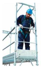
40 • erecting 1st level side fencing
