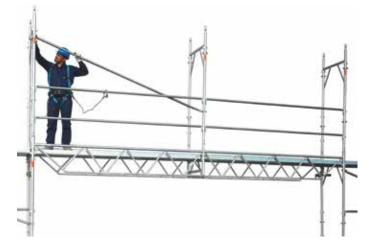
69 • erecting the vertical-diagonal brace above the carriage beams
