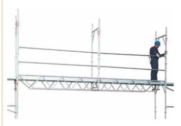
68 • erecting frames and transoms above the carriage beams
