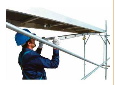
21 • inserting the ladder of the plank with trapdoor
