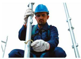
29 • erecting frame pins
