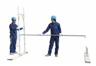
4 • inserting the ledger
