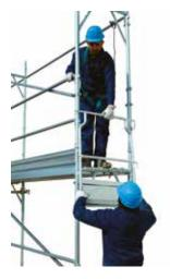
39 • erecting 1st level side fencing
