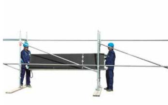
18 • erecting plank with trapdoor
