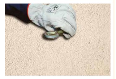
14 • inserting the anchorage
