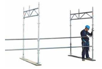
63 • erecting the connections of the pedestrian walk-through frame
