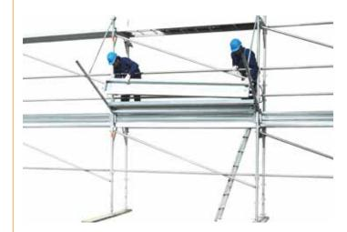
56 • erecting street protection guard planks
