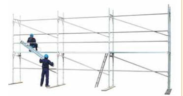
35 • erecting the level 1 toeboard
