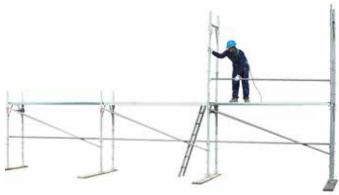
30 • erecting the level 1 ledger
