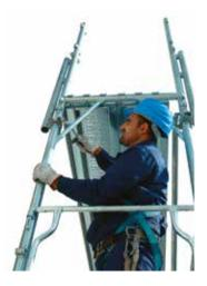
48 • erecting top upright joint on level 2
