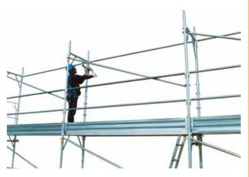
41 • erecting an anchorage on level where needed
