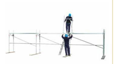
26 • start of frame erection of level 1
