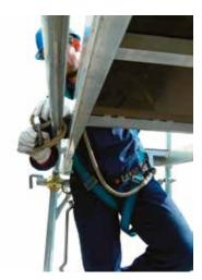
24 • attaching the holding cable before mounting the bay
