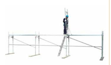
27 • erecting level 1 frame
