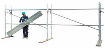
17 • erecting metal ledger boards
