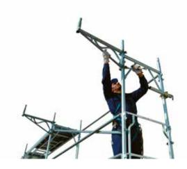
58 • erecting bracket brace
