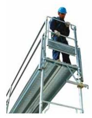
51 • erecting 2nd level side fencing
