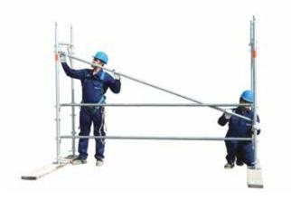
7 • erecting the vertical-diagonal brace
