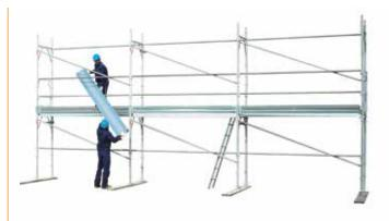
42  $\bullet$  erecting the level 2 planks
