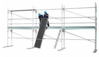
44 • erecting the level 2 planks with trapdoor
