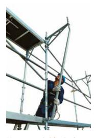
59 • erecting plank bracket brace
