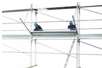
55 • erecting street protection guard planks
