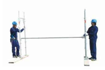
5 • erection second frame with guardrail
