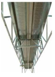
67 • erecting decking on the carriage beam
