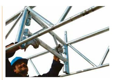
66 • erecting carriage beam connecting beams
